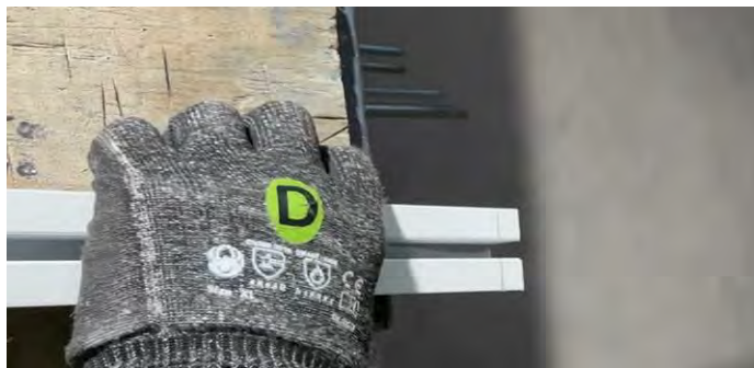
Positioning of the Tate Grid extrusion before coping it
