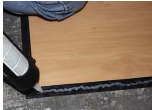
Seam sealer for watertight installation
