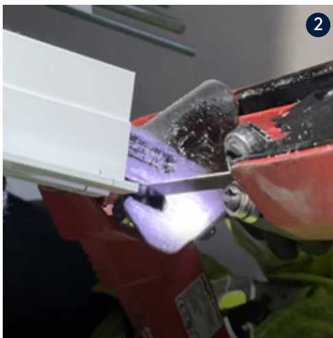
Figure 10.. Field coping with a band saw. Images 2 & 3
