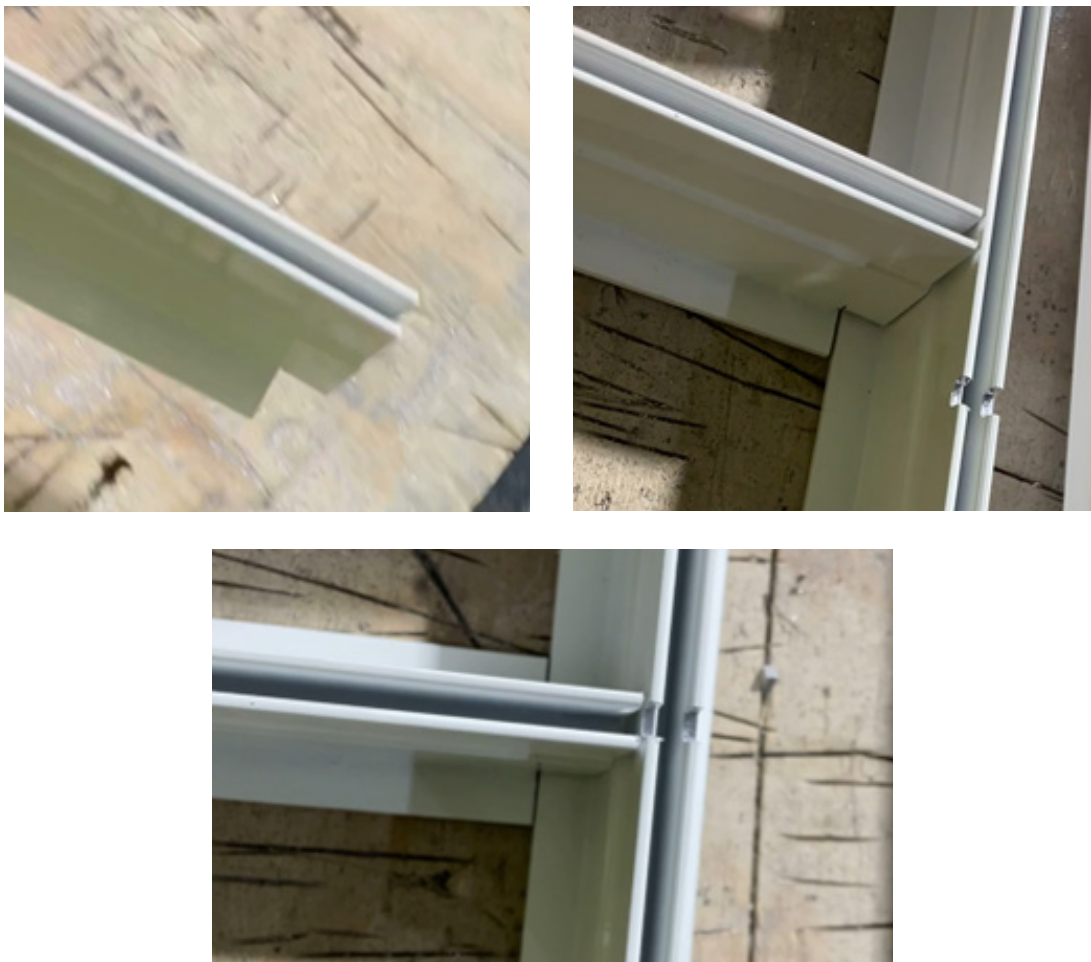
Figure 12. Checking the accuracy of the Field cope
