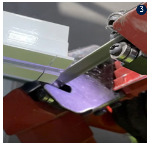
Figure 10.. Field coping with a band saw. Images 2 & 3
