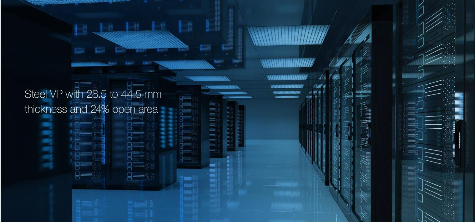
Steel VP with 28.5 to 44.5 mm thickness and 24% open area
