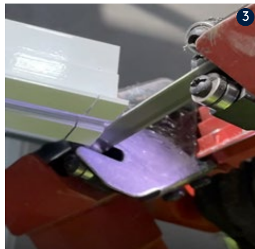
Figure 10.. Field coping with a band saw. Images 2 & 3
