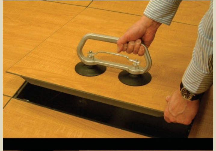
Removing (or reinstalling) a panel with suction cup lifter
